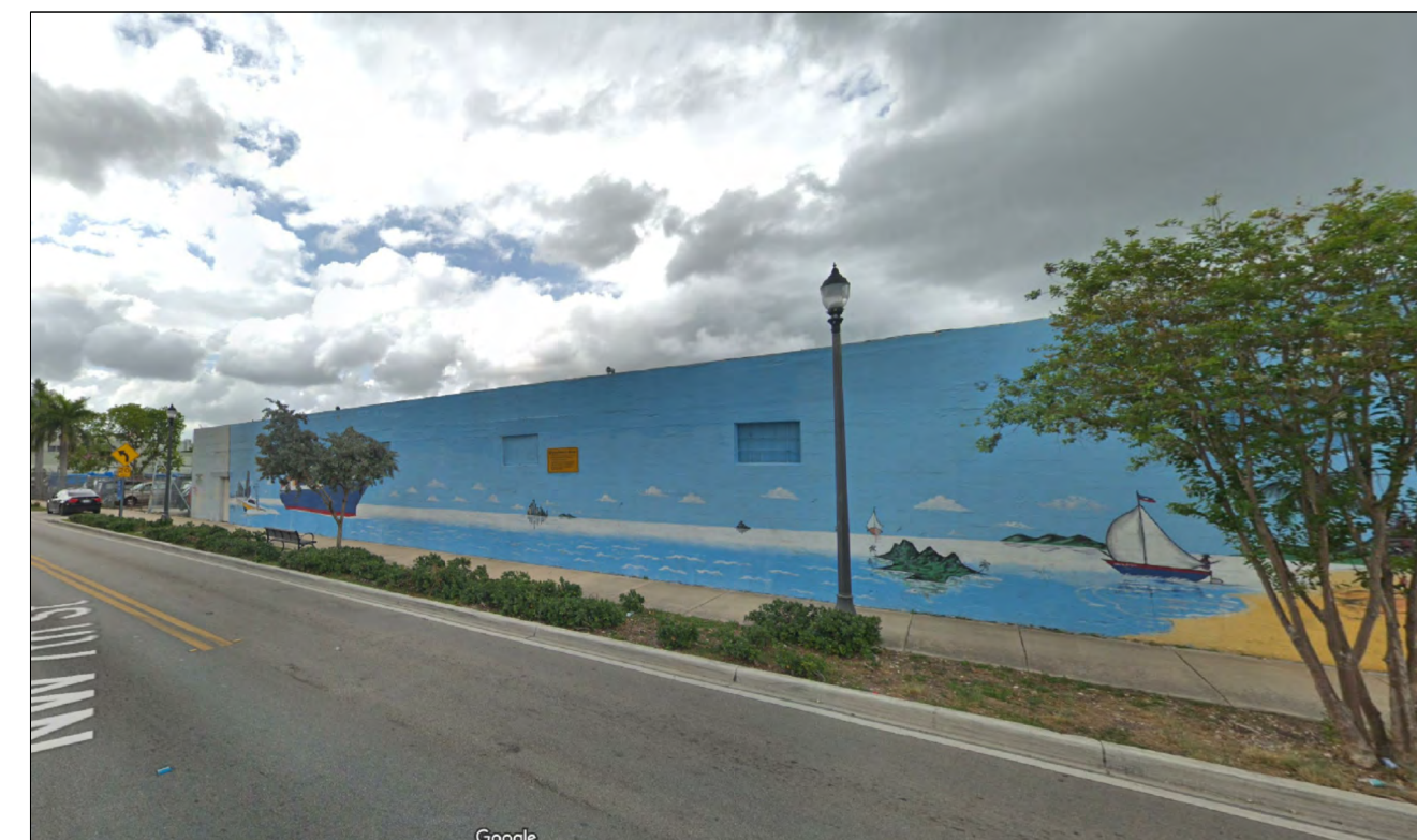
(2) 0 FT EXISTING WALL (631 NW S RIVER DR.)
