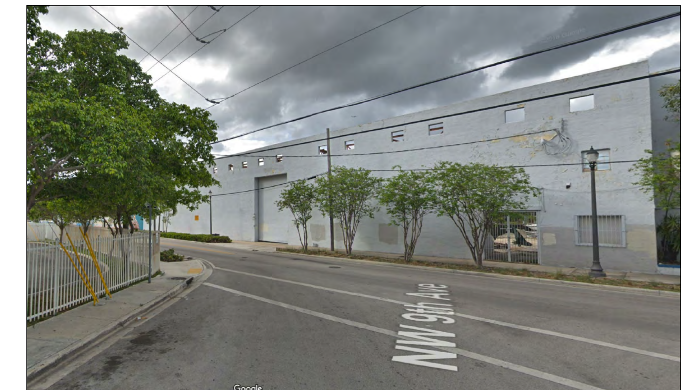
(4) 0 FT EXISTING FENCE (936 NW S RIVER DR.)
