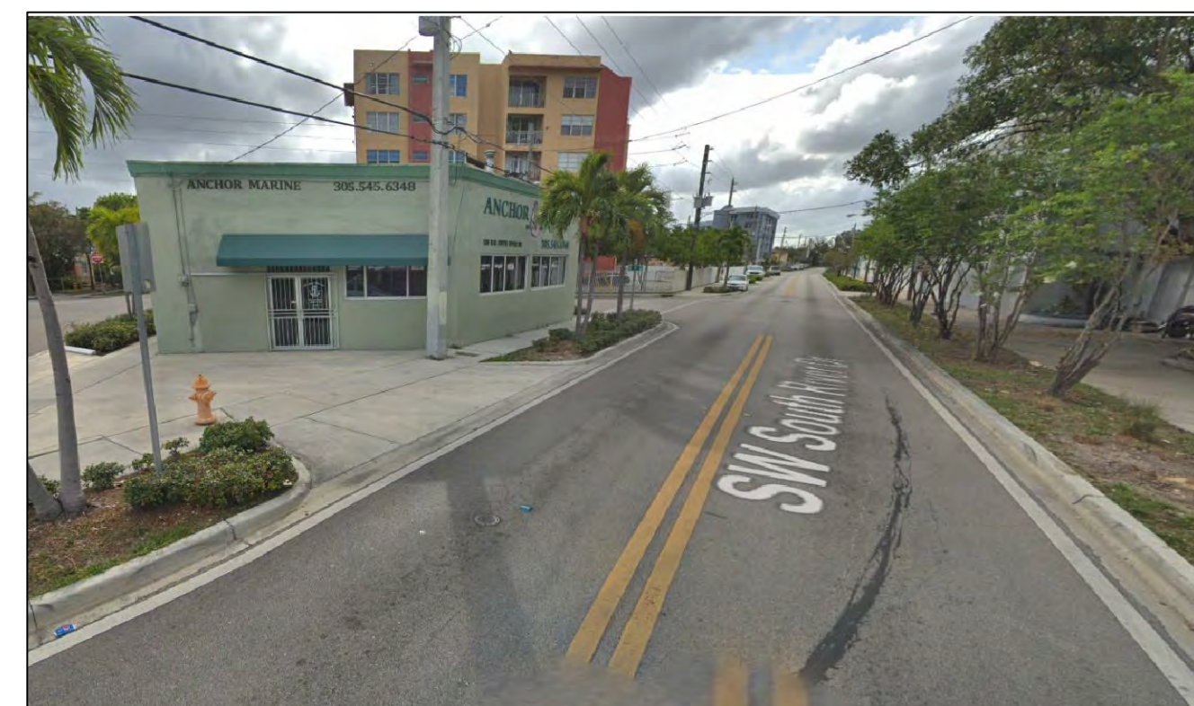
(9) 0 FT EXISTING FENCE (501 NW S RIVER DR.)
